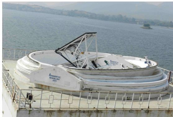
Figure 10: USO's Open (collapsible) Dome
